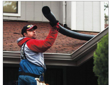
THOMAS PATTERSON | STATESMAN JOURNAL Robert Garza Jr. and workers from ABC Windows install RainTube gutters.
